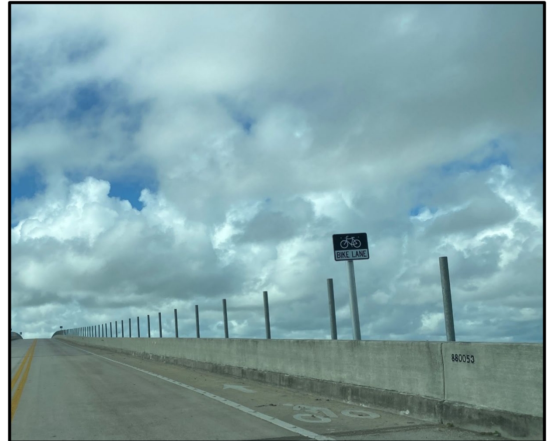
Westbound SR-510/Wabasso Beach Road on the bridge (pre-construction)
