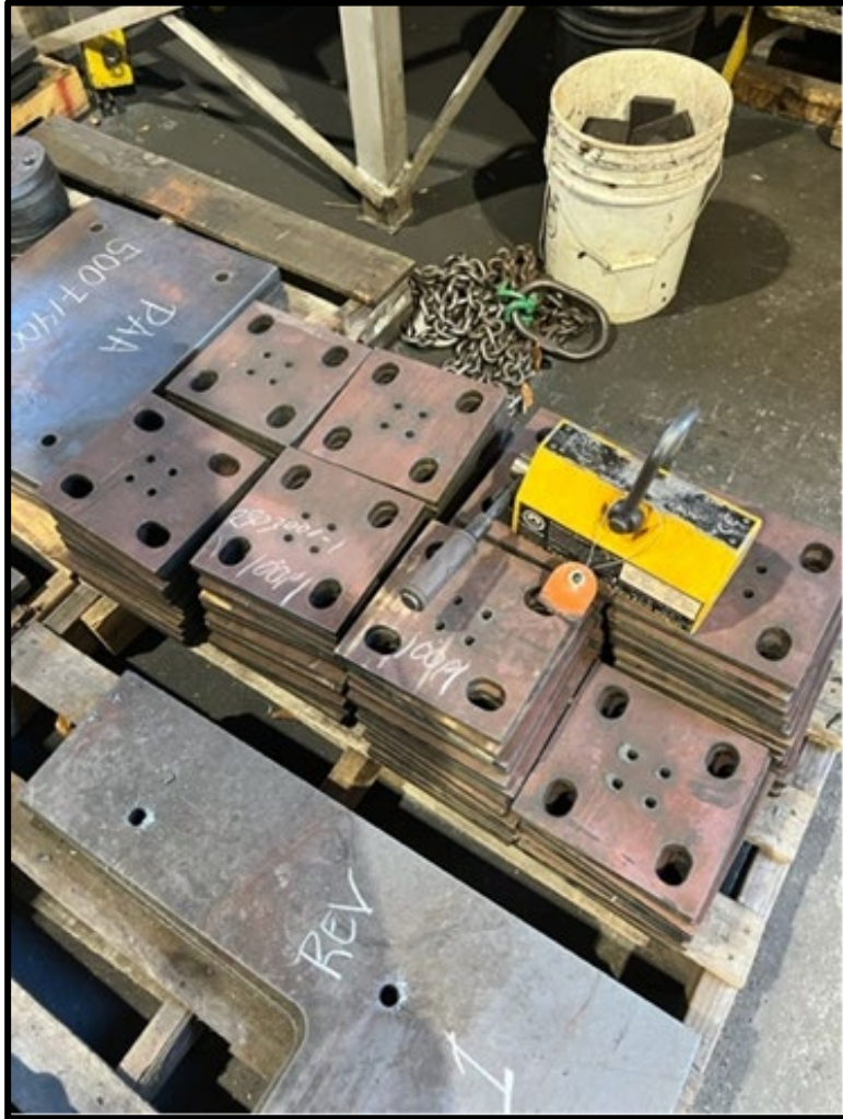
All connection plates and bases have been cut, and connection holes drilled.
