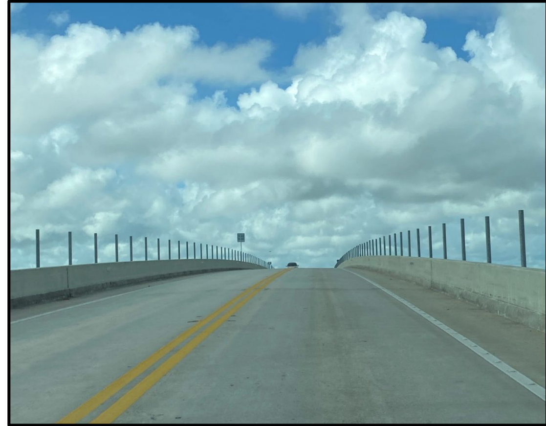
Westbound SR-510/Wabasso Beach Road on the bridge (pre-construction)
