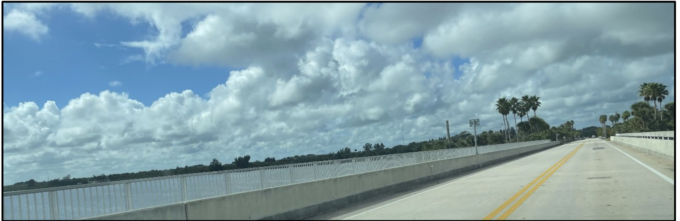
Westbound SR-510/Wabasso Beach Road on the bridge (pre-construction)
